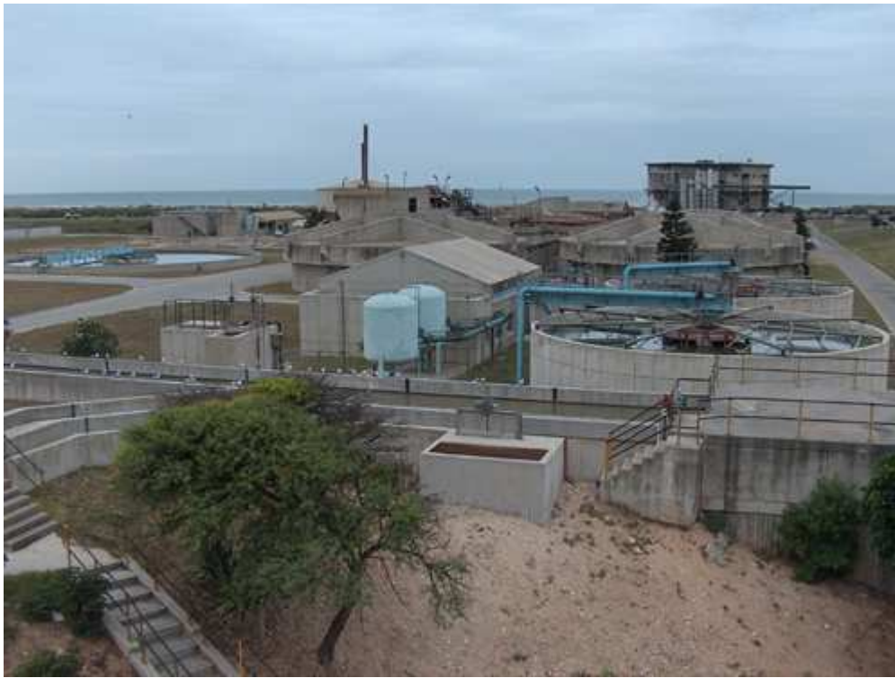
View of Fishwater Flats Sewage Treatment Plant.
