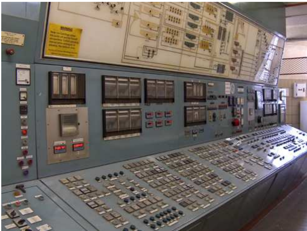
The Existing Mimic Panel soon to be replaced with Computer Based Citect SCADA Mimics and Trend Screens
